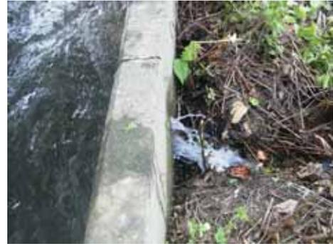
Fig.1 Water leakage from joint part
