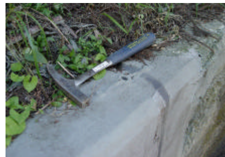
Fig.2 Usual Repair Method of Canal Joint
