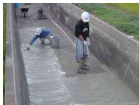
Fig.4 Spraying and Accomplishment
