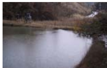
Fig.4 Whole view after earthquake
