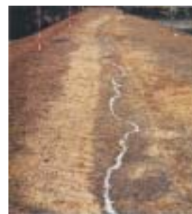
Fig.5 Crack of top surface (After Hyogoken earthquake)
