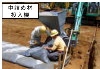
写真-2 中詰め材投入の様子 Filling of soil into soil bag
