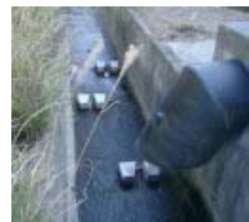
Fig.4 減勢工設置状況 Disposition of stilling dikes
