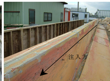
Photo. 2 頂部の充填状況 Filling of the top
