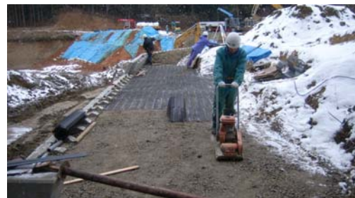
写真-4 転圧 (Photo-4 Compaction)
