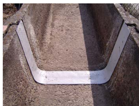
Fig.5 Application of the repair tape
