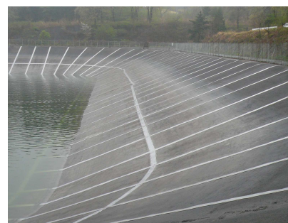
Fig.2 目地部補修後の貯水池 Reservoir repaired of the joint
