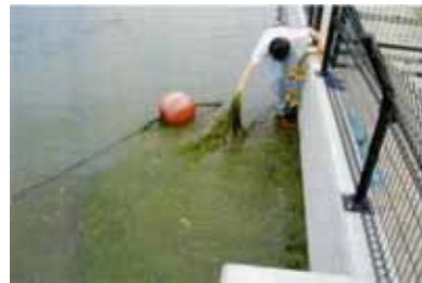
Fig.3 用水路内の水草類の発生事例 Growing of Aquatic Plants in Irrigation Facilities
