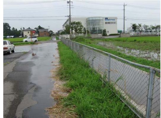
Fig.4 幹線水路からの溢水 Flood from main irrigation canal
