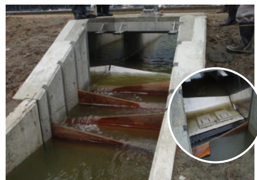
図2 ゲート前面（円内は扉体部分） The front view of gate (A photo in the circle show a float part)
