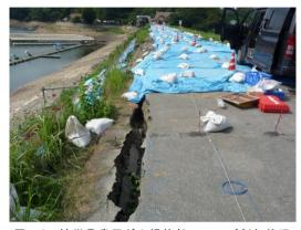
図 - 1 被災農業用ダム提体部でのひび割れ状況 Overview of crack distribution of damaged agricultural dam.
