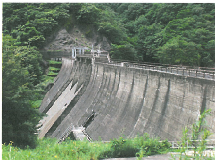
Fig.1 龍生(りゅうい)ダム The view of Ryuui Dam
