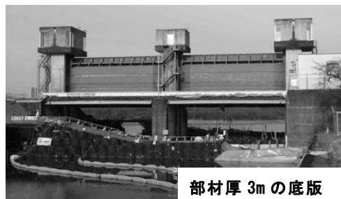
図-6 水門の底版への適用例 / Application for slab of gate
