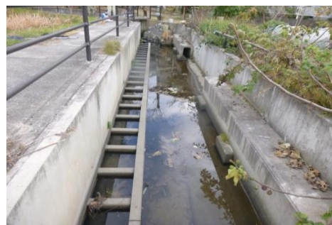
図2. 魚巢と掘り下げが施工されている水路区間 (St. 4). The study station (St. 4) with fish nursery blocks and with deep water depth.
