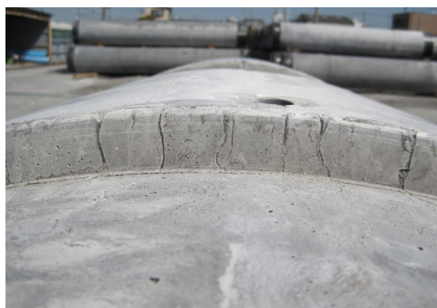
Pic 1 管頂部充填 The filled pipe top
