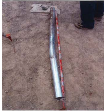
Fig.6 Bending failure of steel pipe after lateral test
