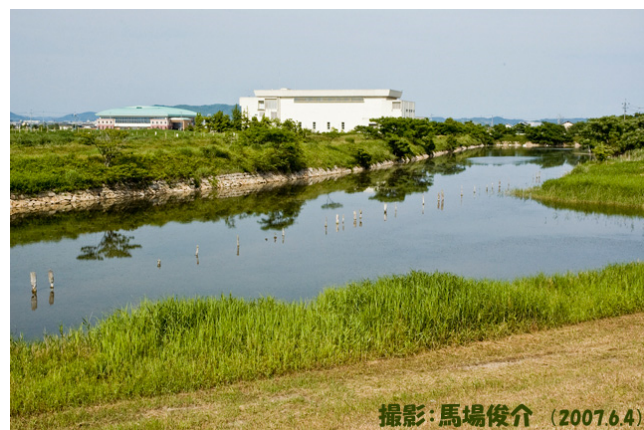
大水尾 (Oomio water storage)
