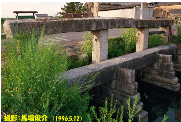
内尾大水門 (Uchio reclamation gate)
