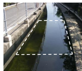
図1 沈砂池の概観 Overview of settling basin
