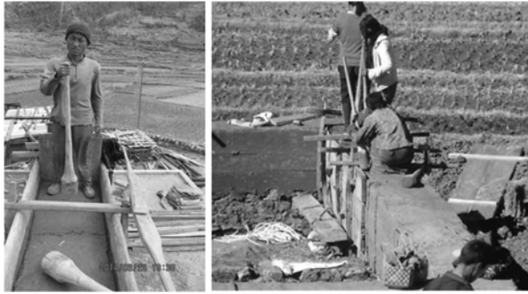
Fig.2 版築工法 Wall making method
