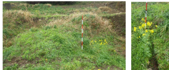
Photo 3 水路埋没地点の地上写真 Pictures of buried channel works recorded on the ground
