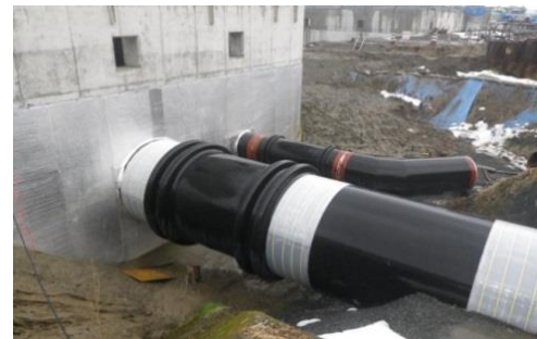
図 1 大変位吸収鋼管 Fig.1 Steel pipe for large displacement
