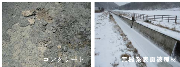
Fig.1 凍害と摩耗を受ける開水路 Open channel exposed to frost damage and abrasion
