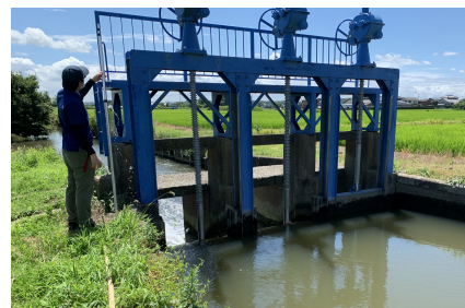
Fig. 1 排水路内の取水堰 Diversion weir in a drainage canal
