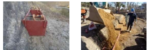
図6 薄層段切り工法施工状況 Construction of thin layer and bench cutting method
