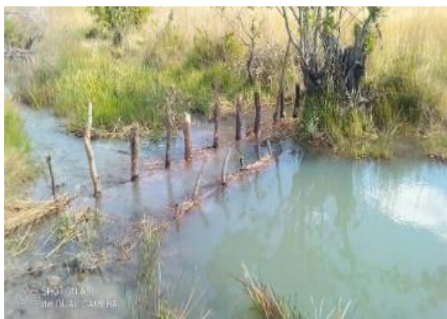
Fig.2 Simple weir submerged by the inflow of rainwater
