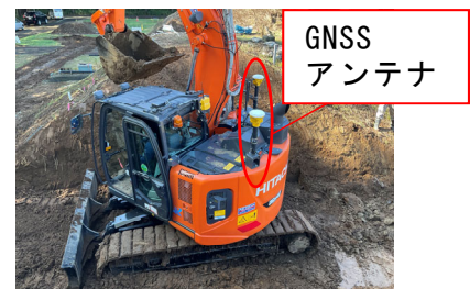
Fig.4 ICT施工状況写真 Photograph of ICT construction
