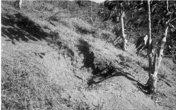
Fig. 8 Silt trap in coffee plantation.
