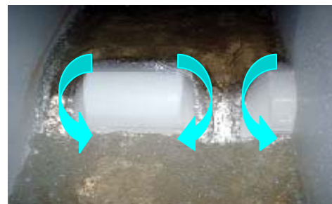
Fig.2 鋼製の曲面スリット部 Curved surface slit department of steelwork
