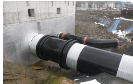
図 2 大変位吸収鋼管 Fig.2 Steel pipe for large displacement
