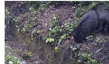
図 4 余水吐に土砂を落とす Soil Dropping down into the Spillway
