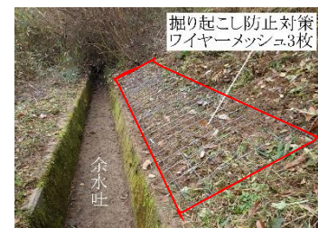
図 6 簡易な掘り起こし防止対策 Easy Countermeasure to prevent Rooting
