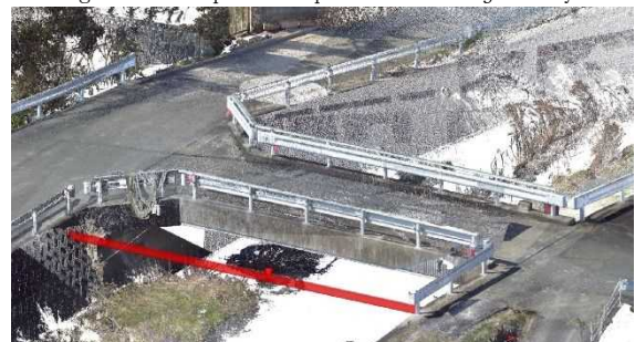
図4 西条市で取得した点群データと施工予定の水管橋 fig.4 Point cloud data acquired in Saijo City and water pipe bridge to be constructed
