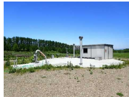
Fig.2 調査対象施設 Facility surveyed
