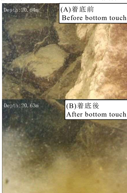
Fig.2 ダム湖底の状況 Condition at the bottom of the dam
